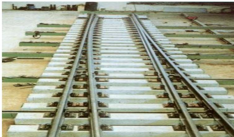
**Figure 1: Concrete sleepers in a siding railway**
